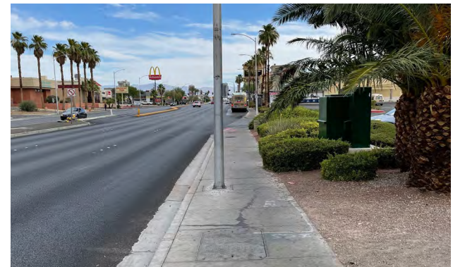
Sidewalk impeded by utility pole
