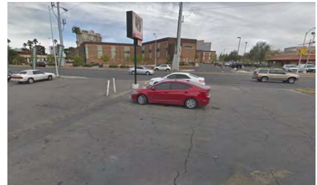
Lack of natural access control
