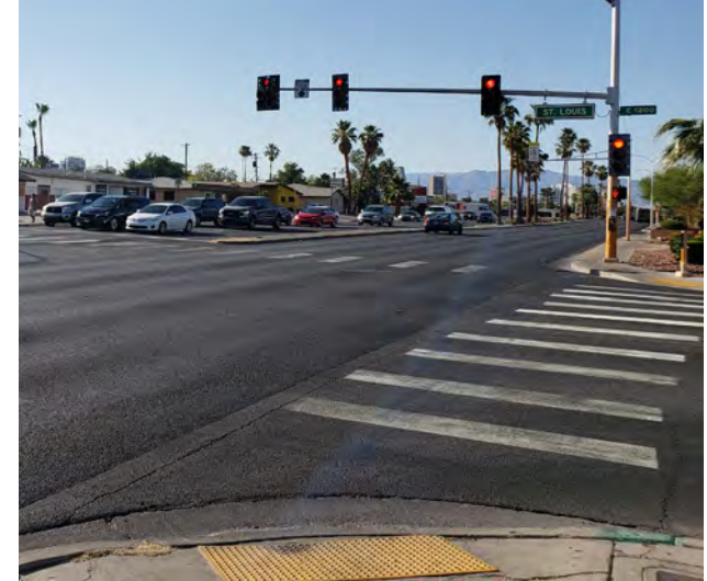
Pedestrian crossings across Maryland Parkway
