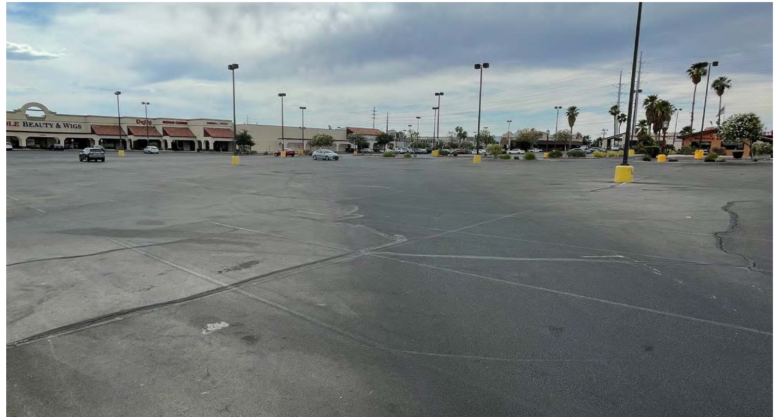
Poor pedestrian connections through parking areas
