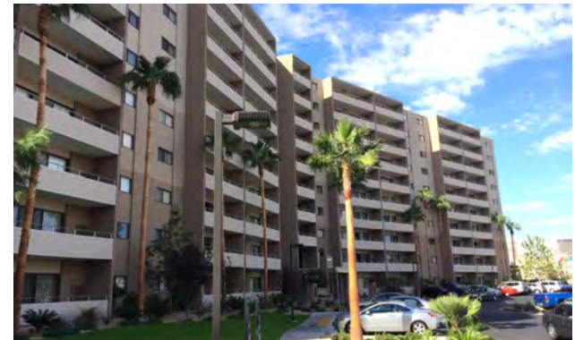
Multifamily high-rise along Flamingo Road
