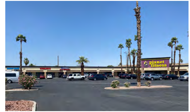
Commercial strip mall and parking
