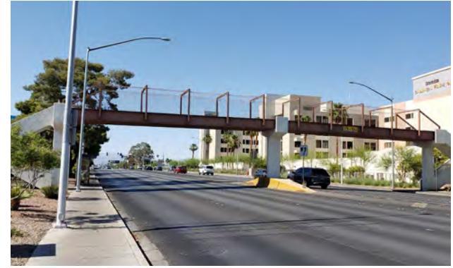
Sunrise Hospital pedestrian bridge
