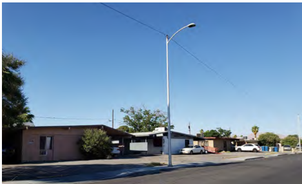
Lighting in residential neighborhood
