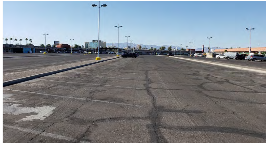
Lack of pedestrian connections through parking areas
