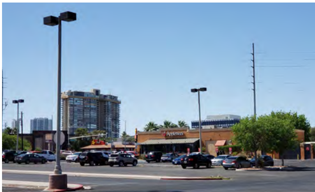
Parking lot with lighting
