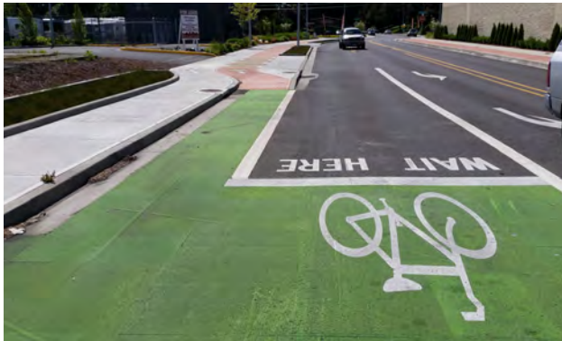
Bike boxes provide designated space at signals
