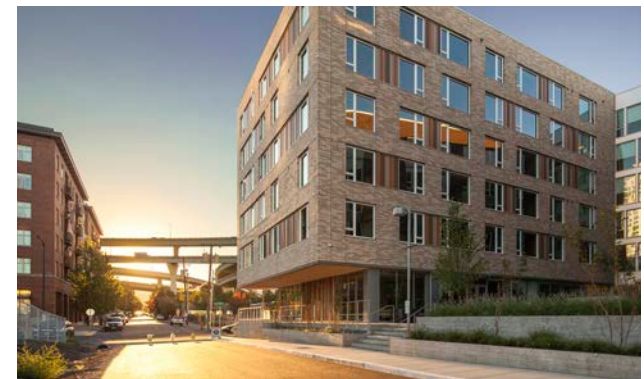
Larger scale, well-coordinated developments can support both market rate and affordable units
