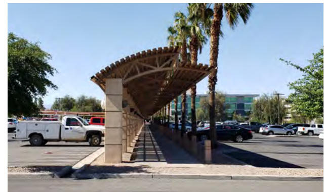
Covered pedestrian walkway near Sunrise Hospital
