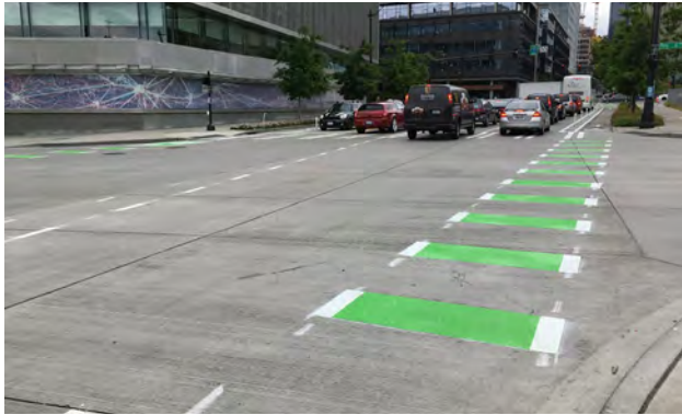
Bike crossing markings through an intersection
